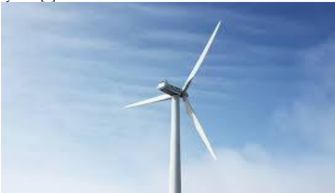
Figure 1.2: Wind Turbine Assembly
